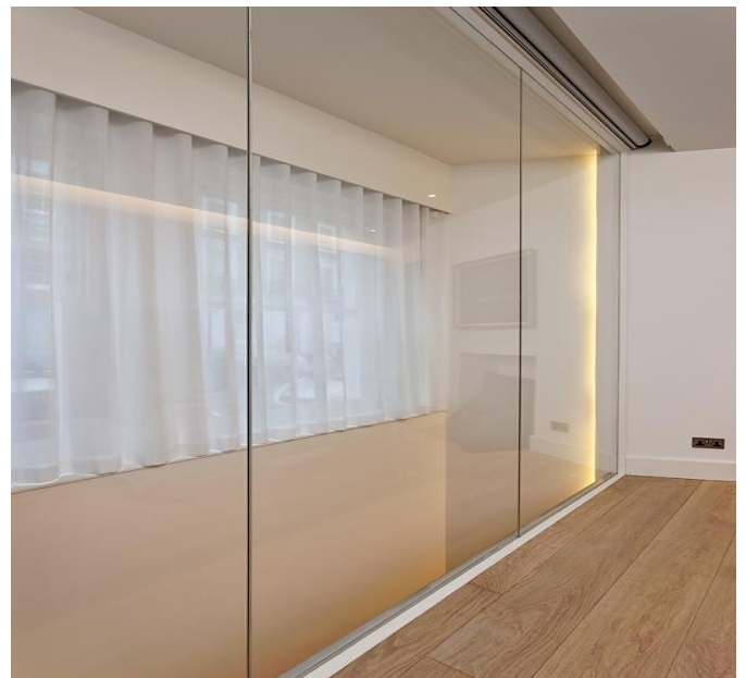
Pyrovista® Butt Joint Glazing System installed in Notting Hill, London Project Architects Haines Phillips
