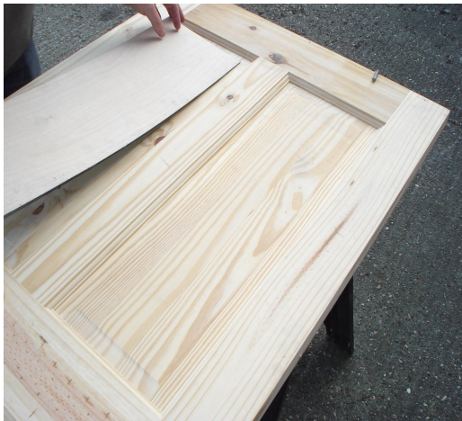
Pyroplaque being applied to thin door panels
